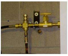
20" header length (Header pictured above accommodates 2 - 72" flexible pigtails for 2 portable bulk vessels + relief valve with pipe away)
