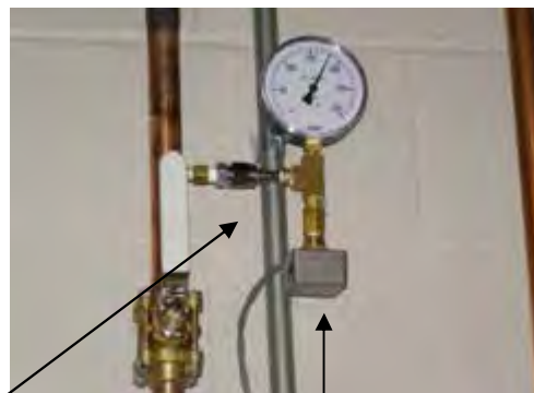
Knock out for low voltage—remote alarm wiring
