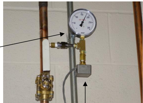
Knock out for low voltage remote alarm wiring
