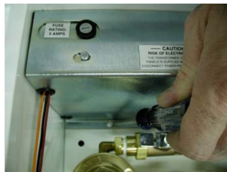
Conduit knockout for low voltage alarm signals
